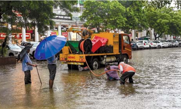
NDMC workers carry out drainage work on a waterlogged road amid rain at Connaught Place in New Delhi on Tuesday
