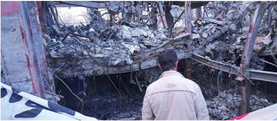
A man looking at a destroyed building within the Grand Hosseiniyeh complex in Zanjan, Iran
