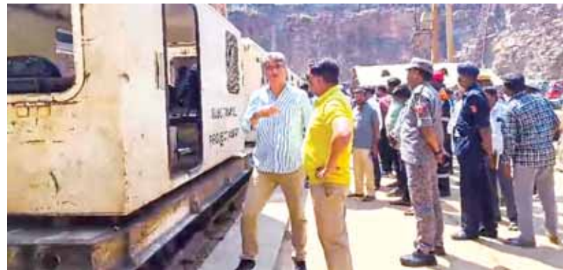
Rescue operation underway to trace workers trapped inside SLBC tunnel in Nagarkurnool
