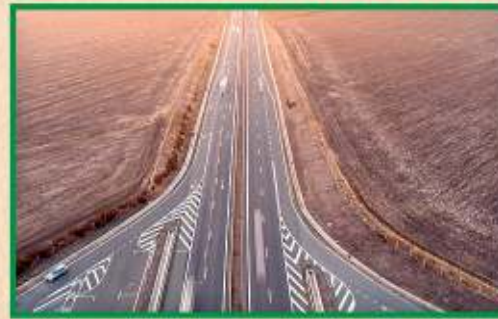
234.28 km of Roads (7 Projects) - ₹ 3,044 Cr
