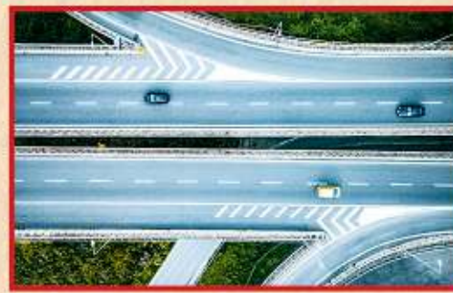
Road Construction/Expansion (10 Projects) - ₹ 4,593 Cr
