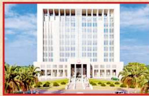
Construction of Visakhapatnam Railway Zone Headquarters - ₹ 149 Cr
