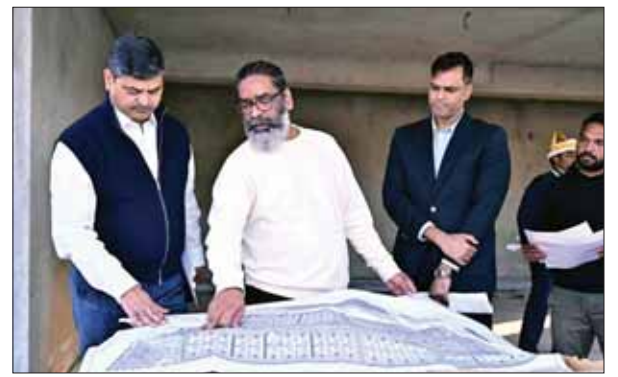
Chief Minister Hemant Soren inspecting the under-construction MLA residential complex, Jagannathpur, Ranchi, including MLA residence, health centre, shopping complex and other construction works, in Ranchi on Wednesday. PNS
