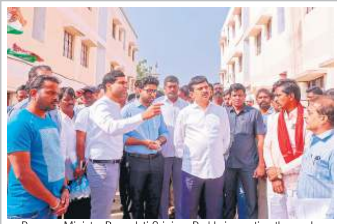
Revenue Minister Ponguleti Srinivas Reddy inspecting the newly constructed double-bedroom housing complex at Mallemadugu under Khammam Urban mandal on Saturday
