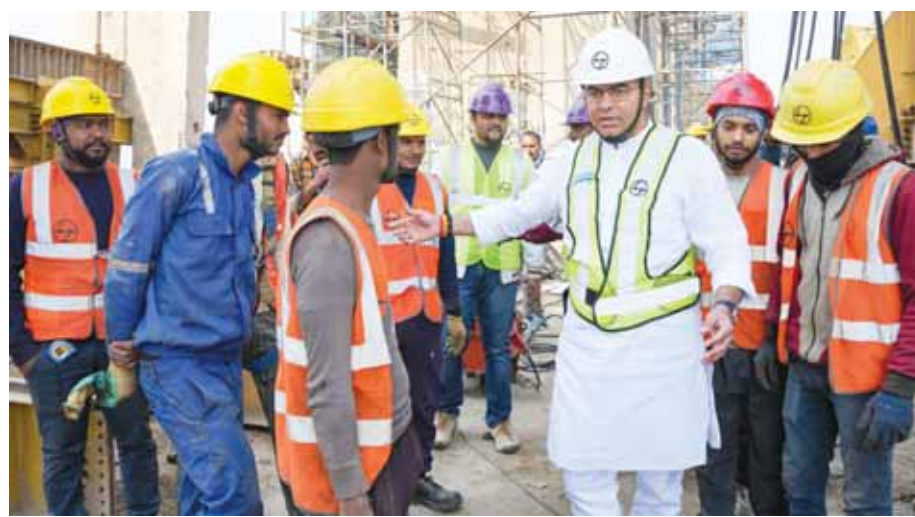
Delhi Deputy Chief Minister Parvesh Verma with workers during the inspection of the Barapullah elevated road project that connects Mayur Vihar to Sarai Kale Khan in New Delhi
