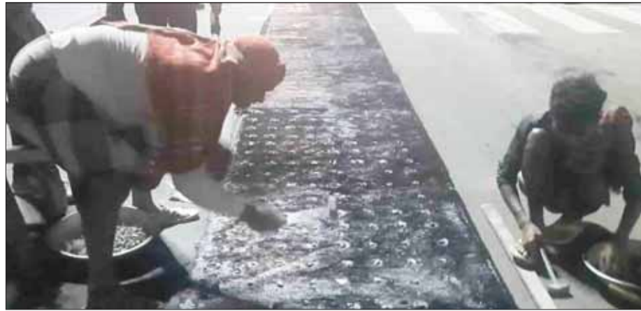
stone mastic asphalt use
