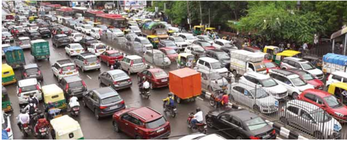
Khanpur metro work led to traffic jam from Panchsheel to the Sheikh Sarai road amid monsoons in New Delhi on Thursday
