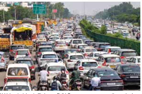
Vehicles stuck in a traffic jam on Delhi-Gurugram expressway as the service lane is closed due to construction work of the underpass between Rajokari (Delhi) to Sirhaul Border
