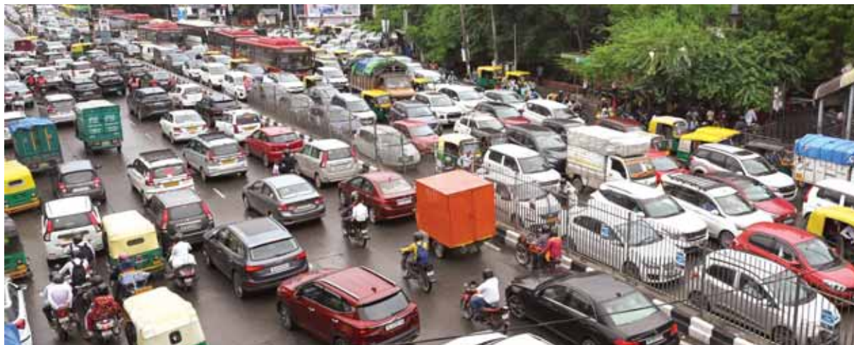
Khanpur metro work led to traffic jam from Panchsheel to the Sheikh Sarai road amid monsoons in New Delhi on Thursday Ranjan Dimri/Pioneer
