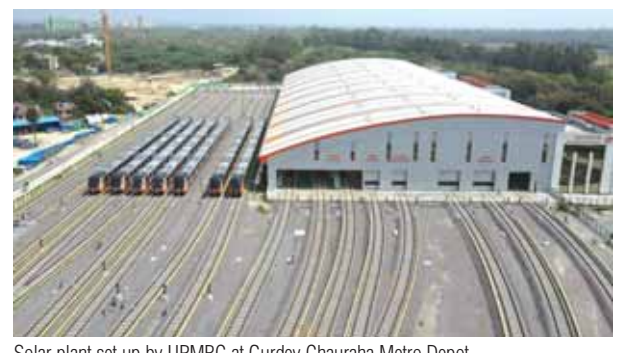
Solar plant set up by UPMRC at Gurdev Chauraha Metro Depot.
