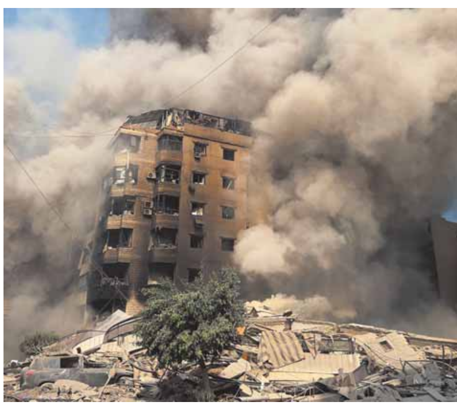
Smoke rises as a building collapses in Beirut's southern suburbs on Saturday.
