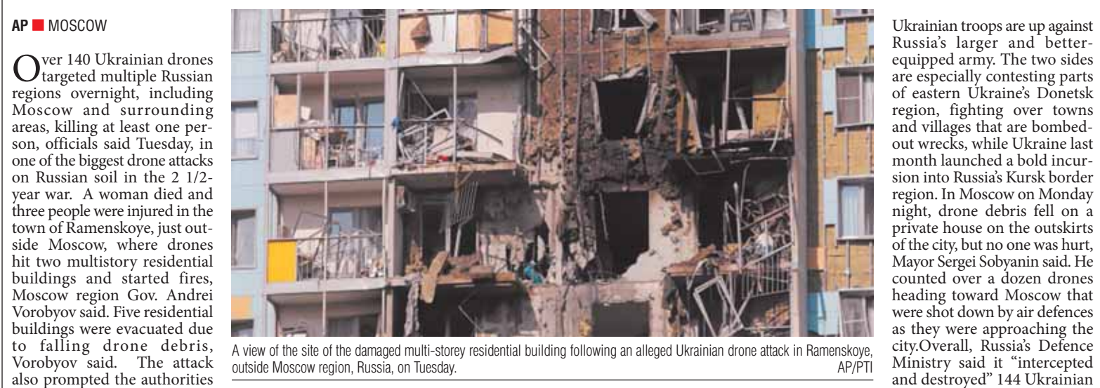
A view of the site of the damaged multi-story residential building following an alleged Ukrainian drone attack in Ramenskoye, outside Moscow region, Russia, on Tuesday.
