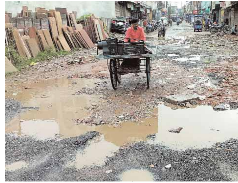
A street washed away following continuous rain in Devki Nagar in Karond locality in Bhopal on Thursday. Pioneer photo
