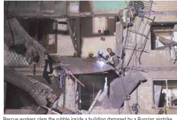
Rescue workers clear the rubble inside a building damaged by a Russian airstrike in Kharkiv, Ukraine, Thursday.
