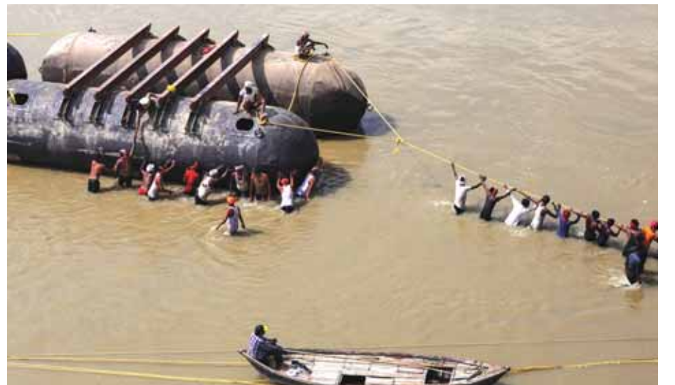
Labourers on Friday build a pontoon bridge on the Ganga river during preparations for the upcoming 'Maha Kumbh Mela' in Prayagraj
