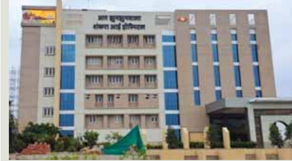
The Sankara Eye Hospital to be inaugurated by PM Modi in Varanasi on October 20.
