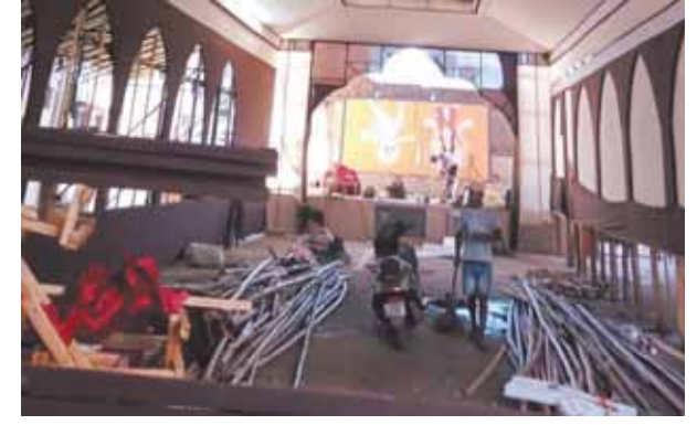
Preparations underway at the puja pandal
