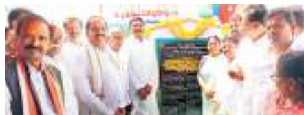
Agriculture Minister Tummala Nageswara Rao at a junction to lay foundation stone for storm drain in Khammam on Thursday
