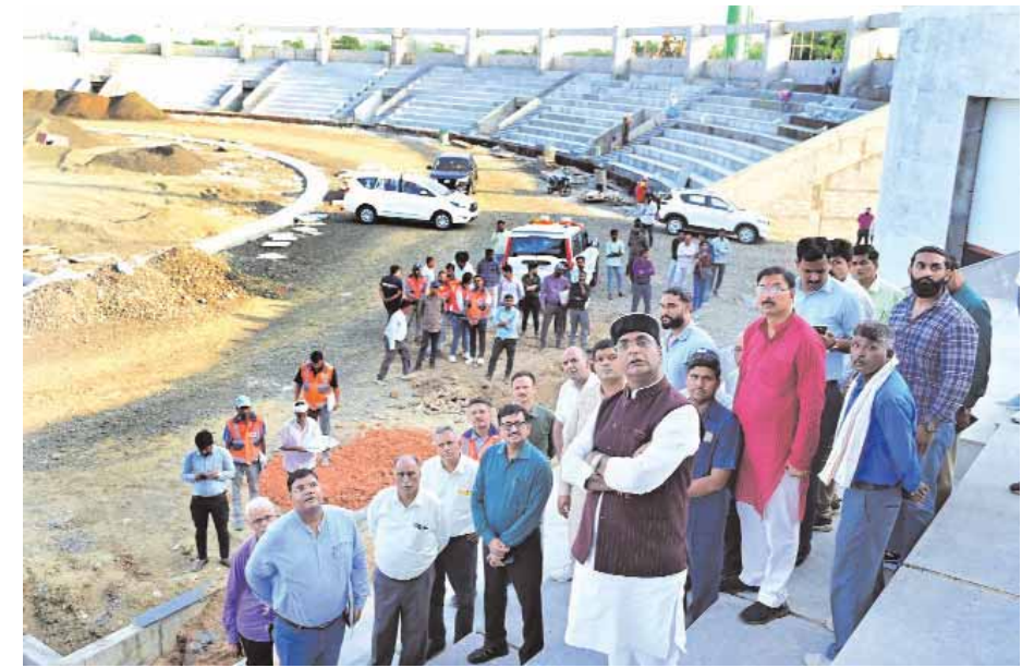
Minister for Sports and Youth Welfare Vishwas Kailash Sarang inspects an under-construction international sports stadium at Nathu Barkheda, on the outskirts of Bhopal on Friday. Pioneer photo
