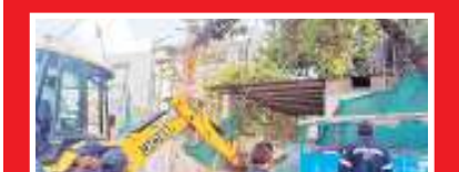
An earthmover dismantling encroachments at Film Nagar in Hyderabad on Saturday
