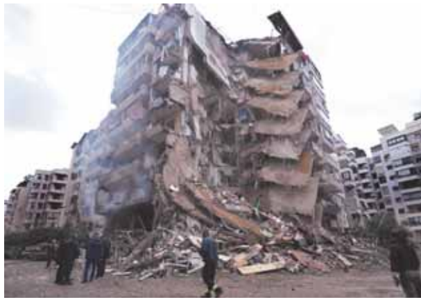
Residents gather in front of a destroyed building that was hit Sunday night in an Israeli airstrike in Dahiyeh, in the southern suburb of Beirut, Lebanon
