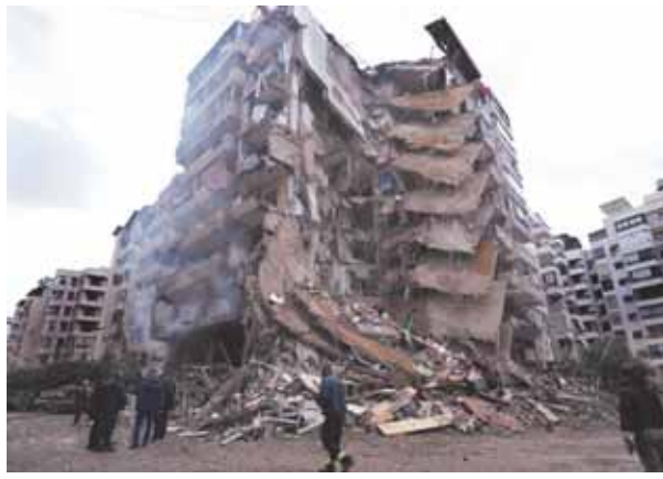
Residents gather in front of a destroyed building that was hit Sunday night in an Israeli airstrike in Dahiyeh, in the southern suburb of Beirut, Lebanon
