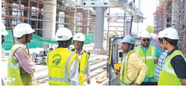
The ongoing work on ropeway project in Varanasi.
