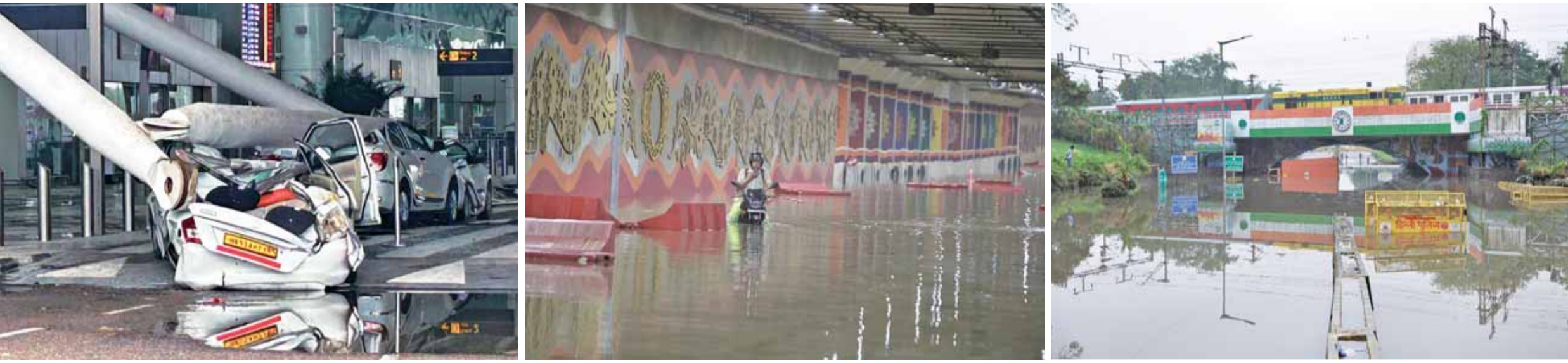
(Left to right): Parked vehicles are damaged by the collapse of a departure terminal canopy at New Delhi's Indira Gandhi International Airport following heavy pre-monsoon rains in New Delhi; Pragati Maidan tunnel underpass waterlogged and waterlogging at the Minto Bridge underpass on Friday Photos: PTI and Ranjan Dimri/The Pioneer
