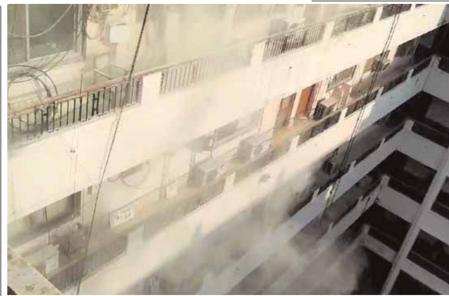
Smoke billows out after fire breaks at State Mantralaya in Bhopal on Tuesday. Pioneer photo
