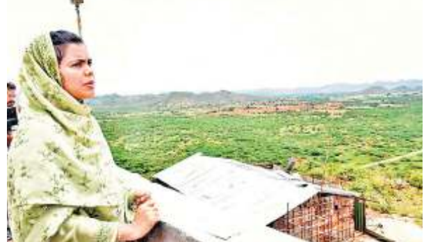
During her inspection of project sites on Tuesday, Collector Ansariya visited affected areas and received updates from officials and engineers on progress. She engaged with villagers in Kalanutala, a submergence village, discussing their concerns such as access to drinking water and basic amenities.
