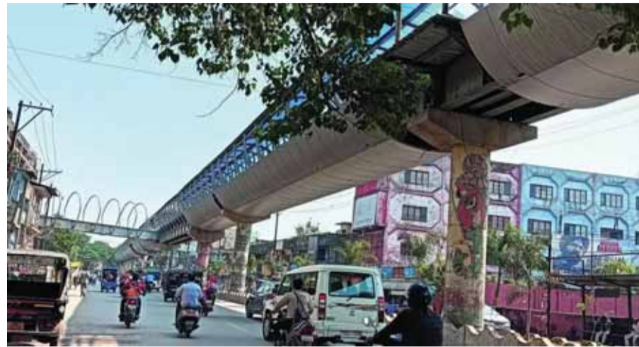
Collector and the work will be taken forward by testing the compensation and the need for land for road widening work between Sharda Chowk and Tatyapara Chowk. The skywalk was needed to facilitate pedestrians on one of the busiest routes between Shastri Chowk and Dr Bhim Rao Ambedkar Hospital Chowk in Raipur.
