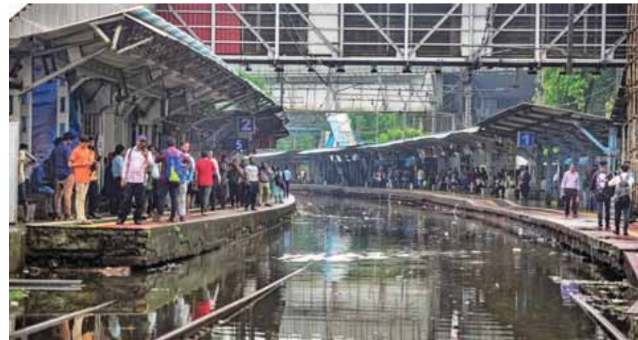
Passengers wait for trains at a waterlogged railway station during rain in Mumbai on Monday
