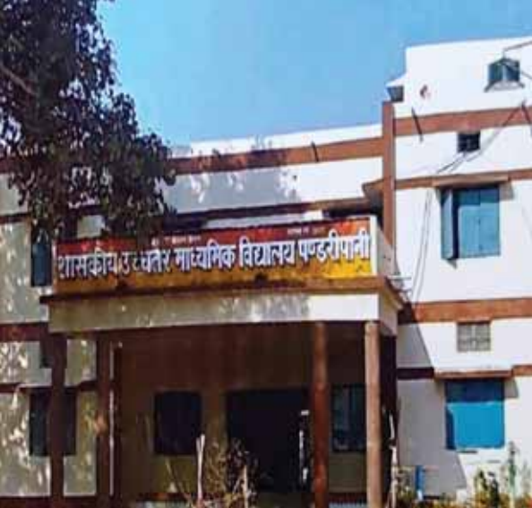
The works include artistic painting, additional rooms, refurbishments and other projects.
