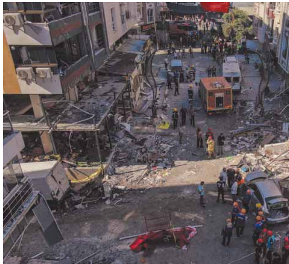
A propane tank explosion at a restaurant in the western Turkish city of Izmir on Sunday left five people dead and 63 others injured, authorities said. Security cameras recorded the explosion, which devastated the street and caused minor damage to surrounding buildings. Interior Minister Ali Yerlikaya announced on social media that dozens of rescue personnel were immediately dispatched to the scene. Izmir Gov. Suleyman Elban visited the injured at the hospital and announced that 40 of them had already been released. Authorities have detained one suspect who might be responsible. The man had replaced the propane tank with a new one on Saturday
