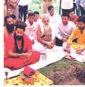
removing encroachment. The corridor will be constructed in almost the same area as the present premises of the temple and the park in front. There are currently two gates to enter the temple. After the construction of the corridor, there will be six gates, then entry will be from Akshayvat Marg. When the devotees leave after bathing in Sangam, they will enter the temple corridor
