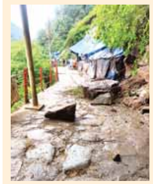
Debris lies on a road following a landslide on the Kedarnath trekking route, in Rudraprayag district, on Sunday. At least 3 pilgrims were killed and several others suffered injuries, according to officials. PTI
