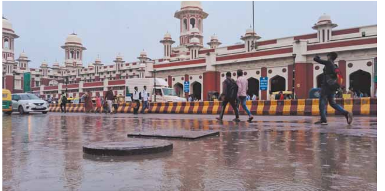
Water accumulated outside Charbagh Railway Station after showers in Lucknow on Wednesday
