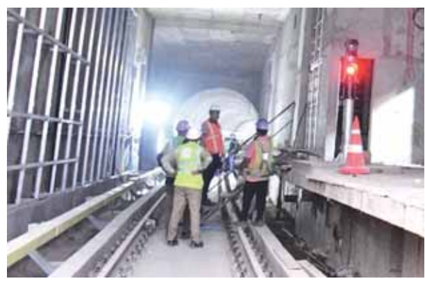
Signal installation at Chunniganj-Nayaganj underground section nears completion.
