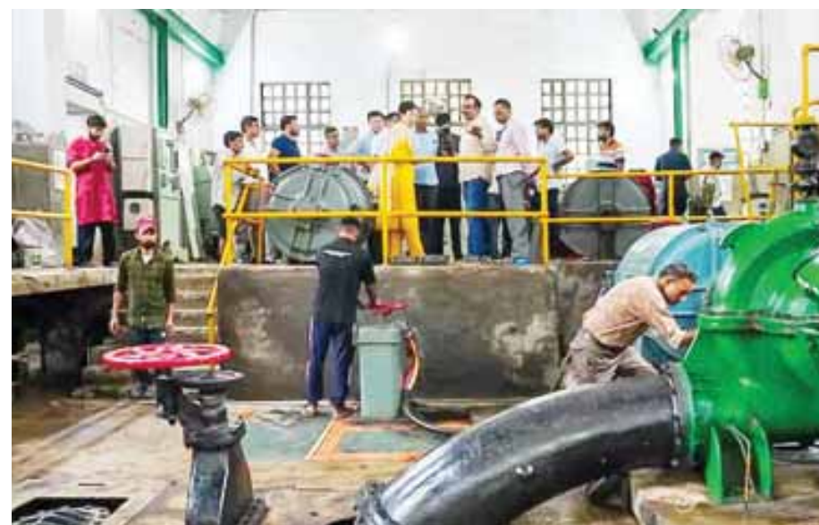
Delhi Water Minister Atishi led an inspection of the Chandrawal Water Treatment Plant's pump house on Sunday morning. "It's noteworthy that Delhi received unexpected rainfall recently. Normally, Delhi receives 800 mm rainfall during the entire monsoon season, but two days ago, 228 mm rainfall occurred in just 24 hours," she said, adding that the water entered the pump house located at Chandrawal Water Treatment Plant. "Due to this, the motors of the pump house had been damaged. Through this pump house, water is supplied to many areas of central Delhi, but due to damage to the motors of the pump house, the supply was disrupted in these areas," she said, adding that the repair of the motors has been completed and the water supply will also become normal. Along with this, Atishi directed the officials that all the concerned departments including Delhi Jal Board (DJB), Urban Development Department to do a joint inspection of the plant and prepare a plan on that basis so that
