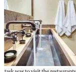
task was to visit the restaurants to identify water-saving potential through simple interventions such as low-flow aerators, which facilitate reducing the flow rate of water from faucets. They achieve this by mixing air into the water stream, which maintains the pressure while using less water.
