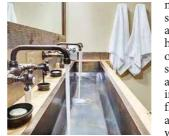
task was to visit the restaurants to identify water-saving potential through simple interventions such as low-flow aerators, which facilitate reducing the flow rate of water from faucets. They achieve this by mixing air into the water stream, which maintains the pressure while using less water. This results in decreased water
