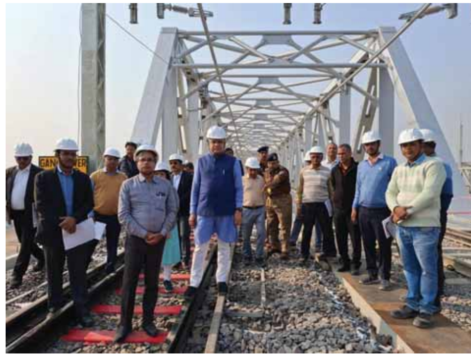
Railway and Information Broadcasting Minister Ashwini Vaishnaw on Sunday inspected the to be commissioned 2.2 kilometres double line New Railway Bridge over Ganga in Prayagraj where the Mahakumbh is scheduled early next year. The Old bridge was single line and of more than 100 years which will be decommissioned shortly. The work for the New Ganga Bridge started in October 2020 and will be commissioned soon by Prime Minister Narendra Modi. Railways also announced that it will run 13000 trains for the Mahakumbh between early January 2025 till February 2025. Pioneer Photo
