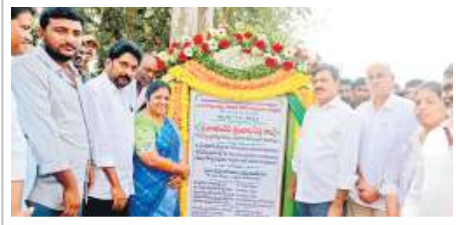
Revenue Minister Ponguleti Srinivas Reddy laying the foundation of the Indiramma Model House at Kalluru in Khammam district on Saturday
