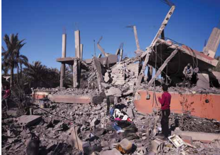
Palestinians check the rubble of a destroyed building following an overnight Israeli strike in Deir al-Balah, Gaza Strip, Wednesday.
