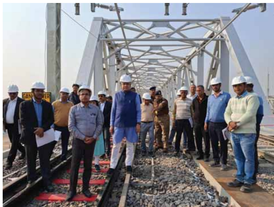
Railway and Information Broadcasting Minister Ashwini Vaishnaw on Sunday inspected the to be commissioned 2.2 kilometres double line New Railway Bridge over Ganga in Prayagraj where the Mahakumbh is scheduled early next year. The Old bridge was single line and of more than 100 years which will be decommissioned shortly. The work for the New Ganga Bridge started in October 2020 and will be commissioned soon by Prime Minister Narendra Modi. Railways also announced that it will run 13000 trains for the Mahakumbh between early January 2025 till February 2025. Pioneer Photo
