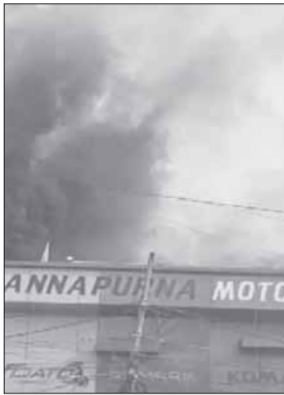
The fire at the electric vehicle showroom in Brahmampur was extinguished after a few hours. The damage to the building and vehicles is significant.
