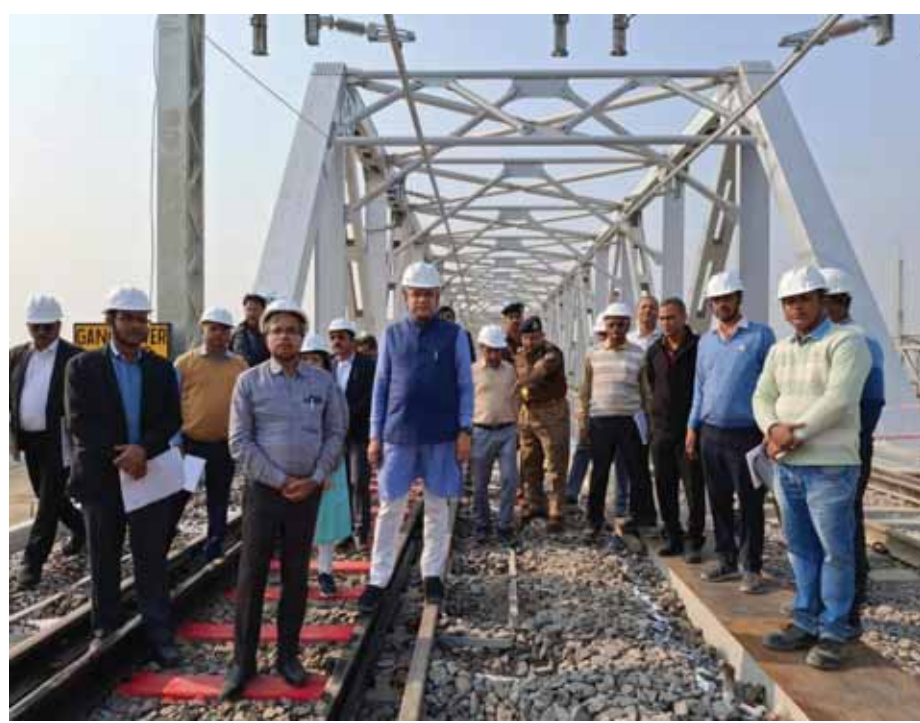
Railway and Information Broadcasting Minister Ashwini Vaishnaw on Sunday inspected the to be commissioned 2.2 kilometres double line New Railway Bridge over Ganga in Prayagraj where the Mahakumbh is scheduled early next year. The Old bridge was single line and of more than 100 years which will be decommissioned shortly. The work for the New Ganga Bridge started in October 2020 and will be commissioned soon by Prime Minister Narendra Modi. Railways also announced that it will run 13000 trains for the Mahakumbh between early January 2025 till February 2025. Pioneer Photo
