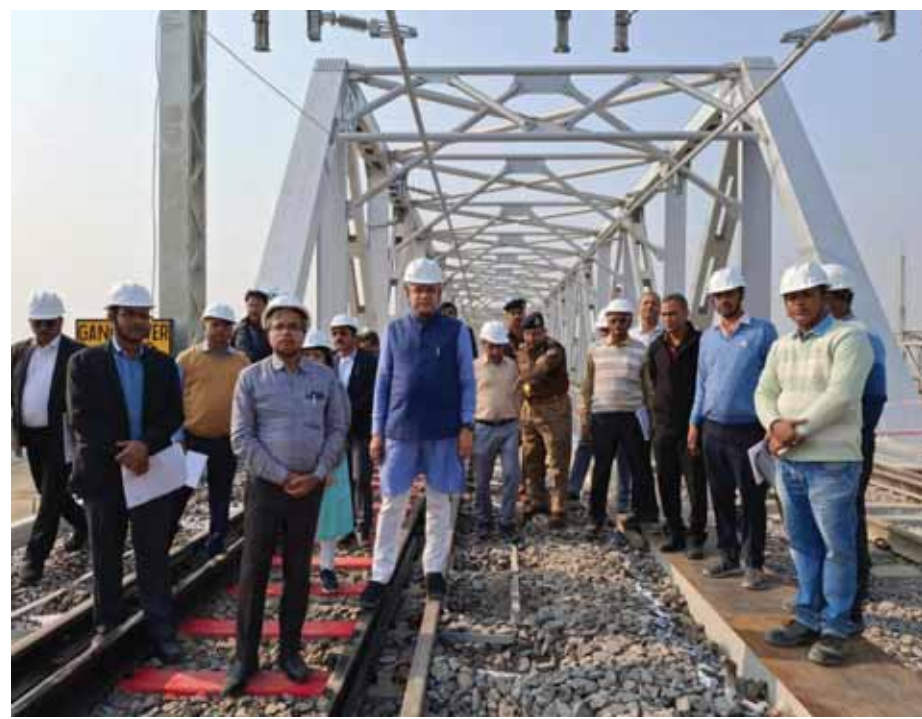
Railway and Information Broadcasting Minister Ashwini Vaishnaw on Sunday inspected the to be commissioned 2.2 kilometres double line New Railway Bridge over Ganga in Prayagraj where the Mahakumbh is scheduled early next year. The Old bridge was single line and of more than 100 years which will be decommissioned shortly. The work for the New Ganga Bridge started in October 2020 and will be commissioned soon by Prime Minister Narendra Modi. Railways also announced that it will run 13000 trains for the Mahakumbh between early January 2025 till February 2025. Pioneer Photo
