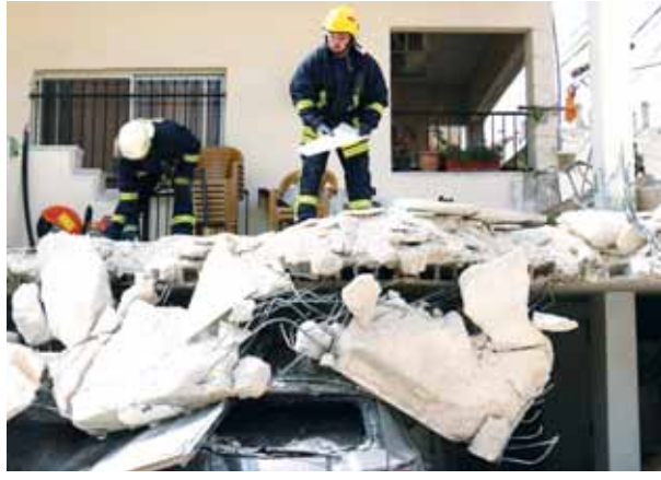
Palestinian civil defense workers clear the rubble from a damaged house following an Israeli military operation in the West Bank refugee camp of Nur Shams, Tulkarem, Friday. AP/PTI
