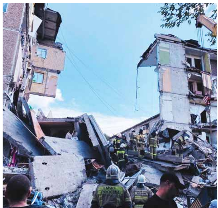
In this photo released by the Telegram channel of the head of Nizhny Tagil Vladislav Pinyavov on Thursday, August 1, 2024, Russian Emergency Ministry workers are seen near a multi-storey building partially collapsed presumably due to gas explosion in Nizhny Tagil, 1400km (870mi) east from Moscow, Sverdlovsk region, Russia. Three people have reportedly been rescued from under the rubble, information about the victims is being clarified AP/PTI
