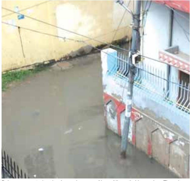
Rain causes waterlogging in a colony near Nagar Nigam in Varanasi on Thursday.
