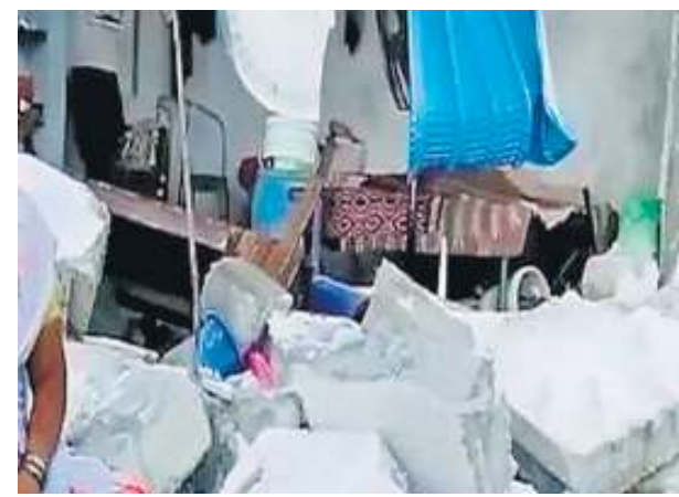
A partly demolished house
